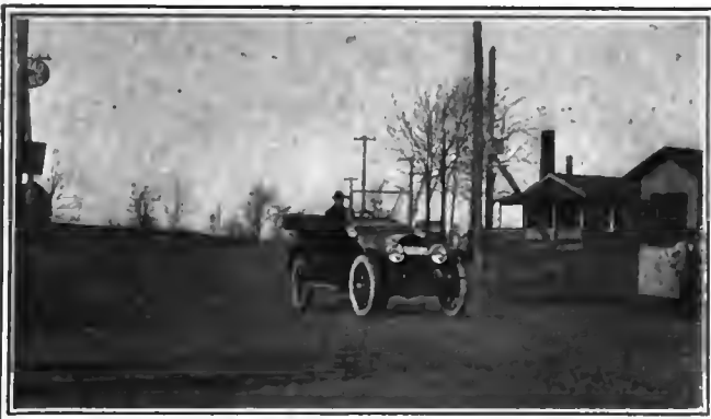
Crossing at Berlin, Conn., where a number of serious and fatal accidents have occurred. Note the absence of gates
